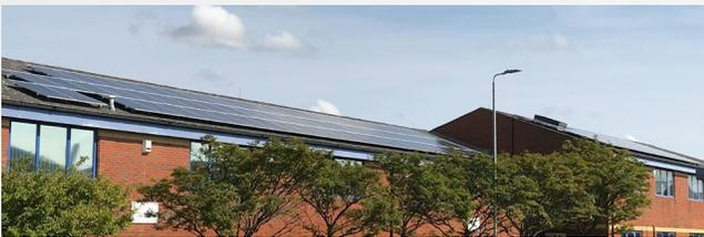
In August 2018 we commissioned a 30 kwh solar roof-top installation, generating approximately 23% of the electricity required to run the NEB UK office and warehouse. Estimated emissions avoided are 21 tonnes of CO<sub>2</sub> per year. The remainder of our power usage is 100% green electricity supplied by Ecotricity.
